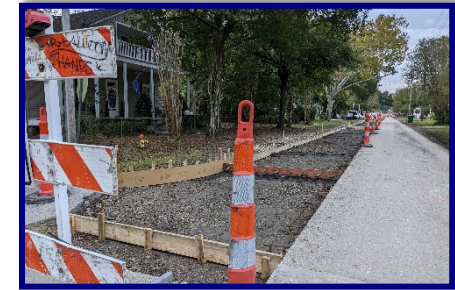
Carey Street Pavement Reconstruction
